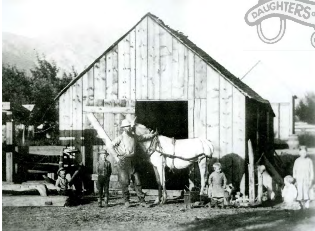
Blacksmith Shop (DUP Photo Collection)
